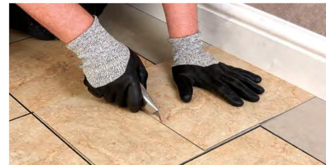
Figure 5.6 Measuring using an overlapping tile
