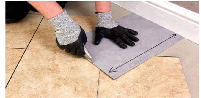
Figure 5.9 Cutting the perimeter tiles (diagonal cut)
