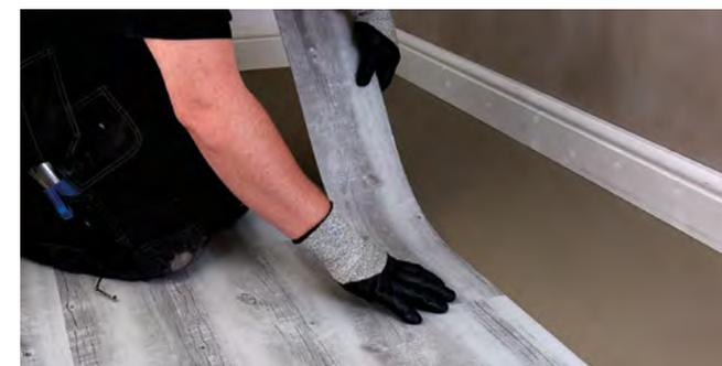
Figure 5.1 Setting planks out
