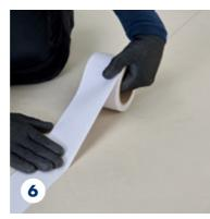
Apply the QuickLay double sided tape along the marked seams.
