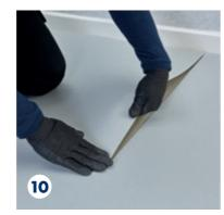
Once complete, place the floor covering into position ensuring a 'neat fit'.
