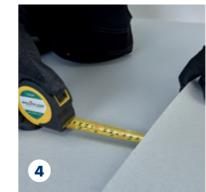
Use the appropriate method to install QuickLay in the room (refer to the relevant section in our Technical Manual). Allow a 25mm overlap at the seams and cut in to form a tight seam.
