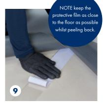
Carefully peel away the protective film from all areas where the tape has been applied.
