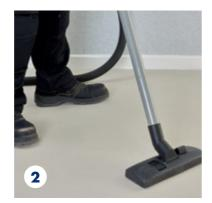
Sweep or vacuum the floor area, check the condition of the subfloor and make good as necessary. If the substrate is highly porous a suitable primer maybe required.
