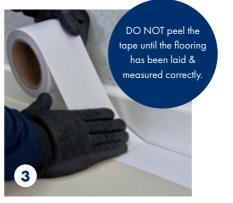
Apply the QuickLay double sided tape around the perimeter of the room and at any doorways, set  $2 \, \rm mm$  away from the edge of the room.
