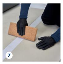
To ensure the QuickLay tape is firmly positioned correctly, simply press down with a hand roller or cork board.
