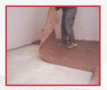
3. INSTALLATION - Adhering DAMTEC® acoustic underlay to substrate.
