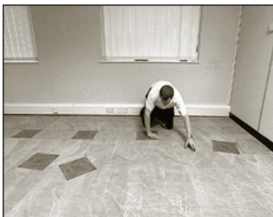
Loose lay tiles to check set out.
