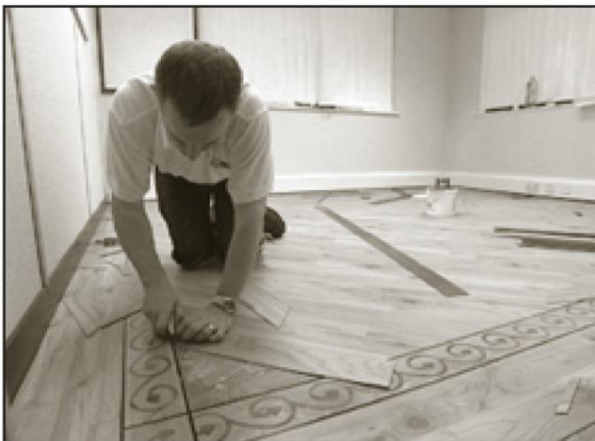
Installing border and perimeter tiles
