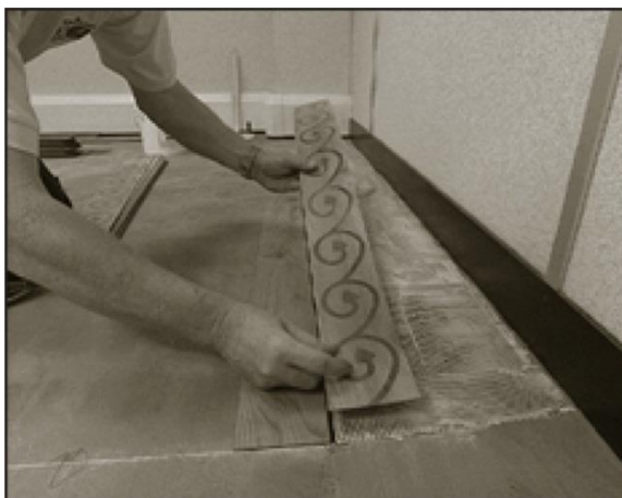
Setting out for border installation
