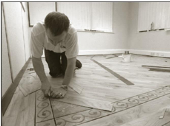
Installing border and perimeter tiles
