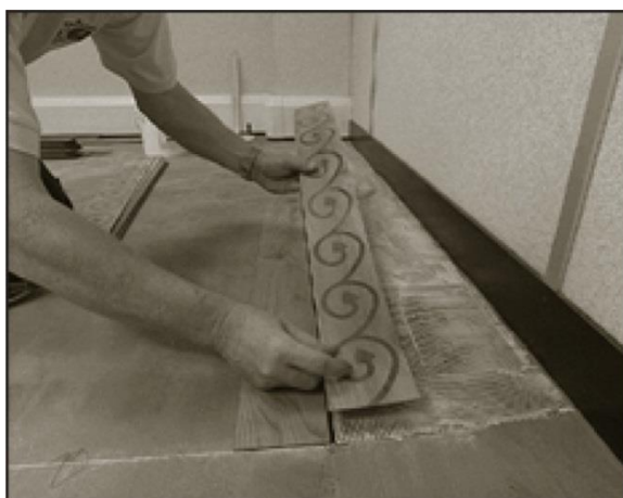
Setting out for border installation
